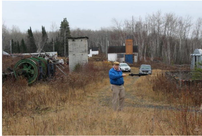
More infrastructure at Tyranite
