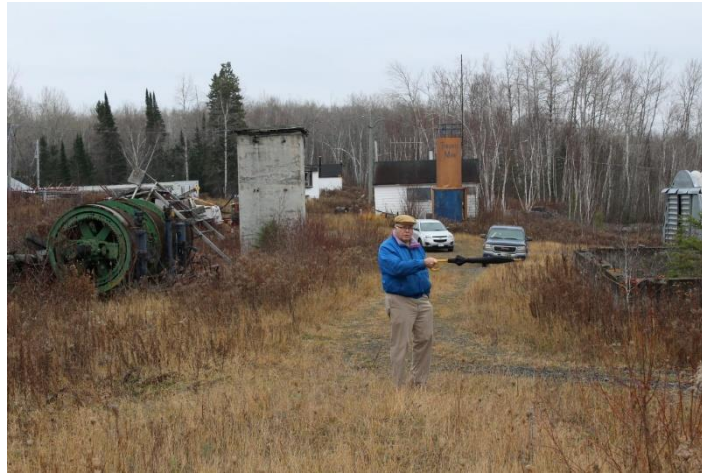
More infrastructure at Tyranite
